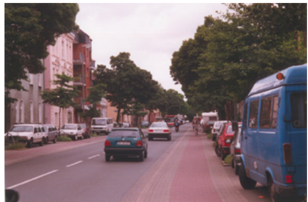
Figure 5B.7 Traffic calming technique of narrowing vehicular lanes and coloring pavement for bicycling and/or parking along pedestrian-oriented streets
